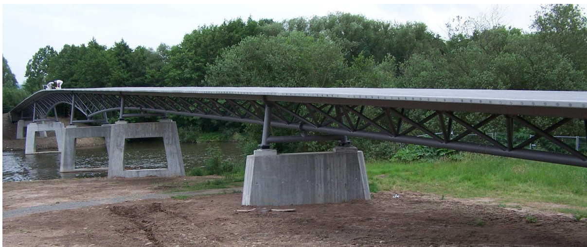
Fig. 1 View of the Gaertnerplatz Bridge in Kassel.
