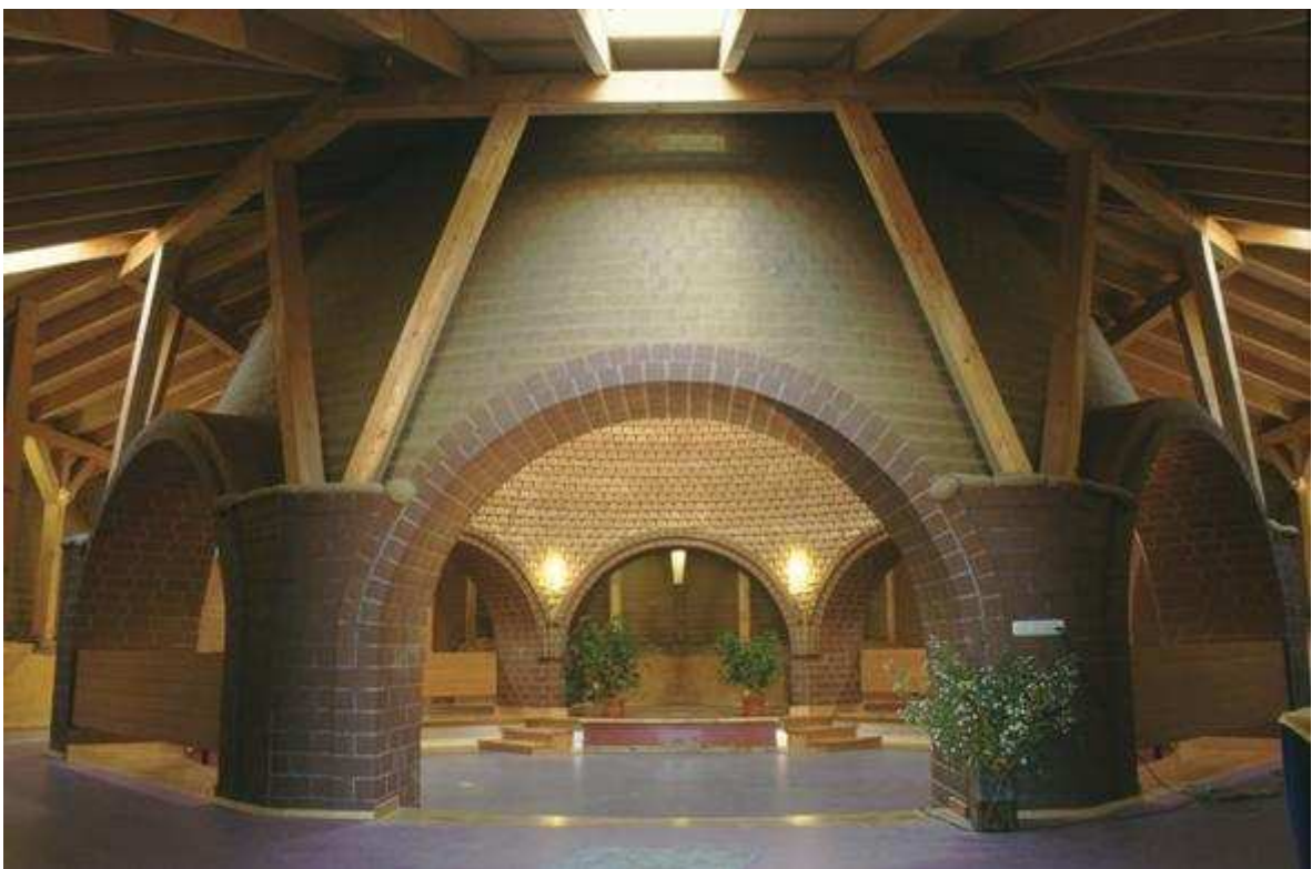
Fig. 18 Multipurpose hall, Kindergarten at Sorsum, Germany
