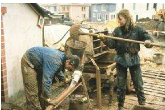
Fig. 15 Interior walls of lightweight loam-filled cotton hoses
