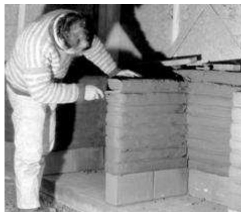
Fig. 14 Extrusion of loam profiles and stacking in a plastic state
