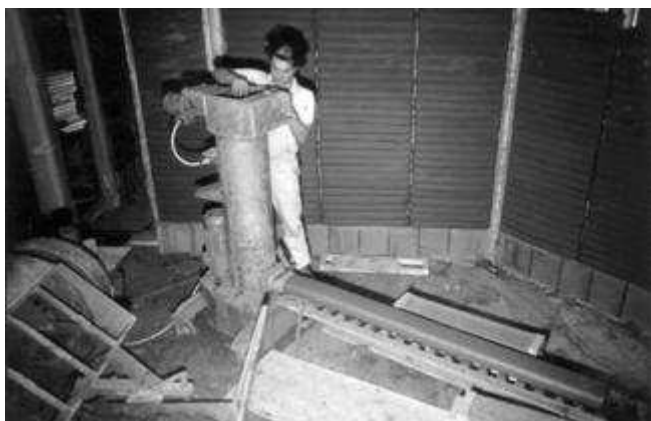
Fig. 13 Extrusion of loam profiles and stacking in a plastic state
