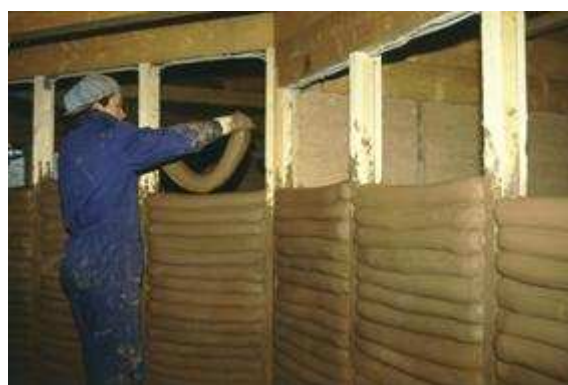
Fig. 16 Interior walls of lightweight loam-filled cotton hoses
