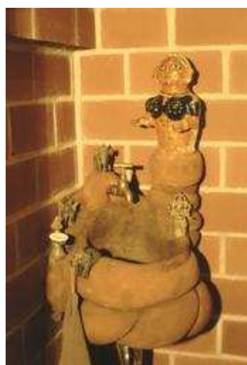
Fig. 9 Wash basins from stabilised loam, residence at Kassel, Germany
