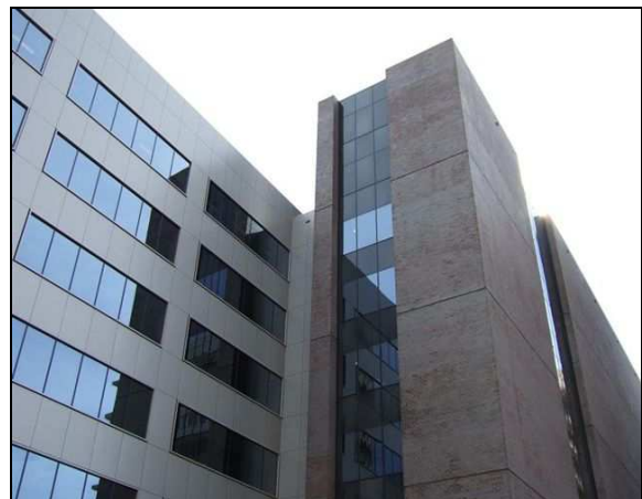
Fig. 1 Centraplaza in Canberra, Australia
