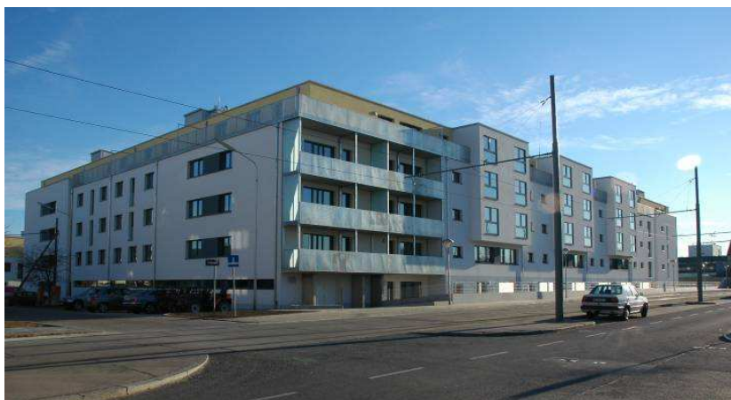
Fig. 3 Residential building “Pantucekgasse”
