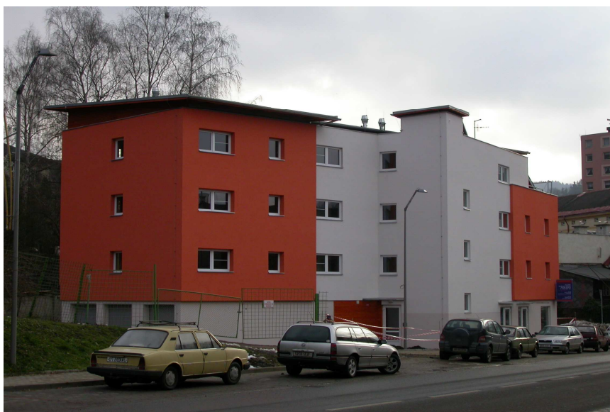
Fig. 3 Apartment house in Železný Brod – main facade
